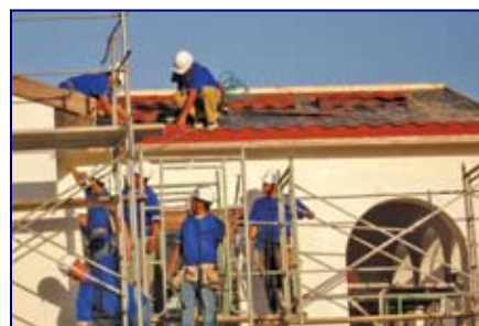
BEFORE shot: Roofing crews begin laying the Barrel Vault panels.
